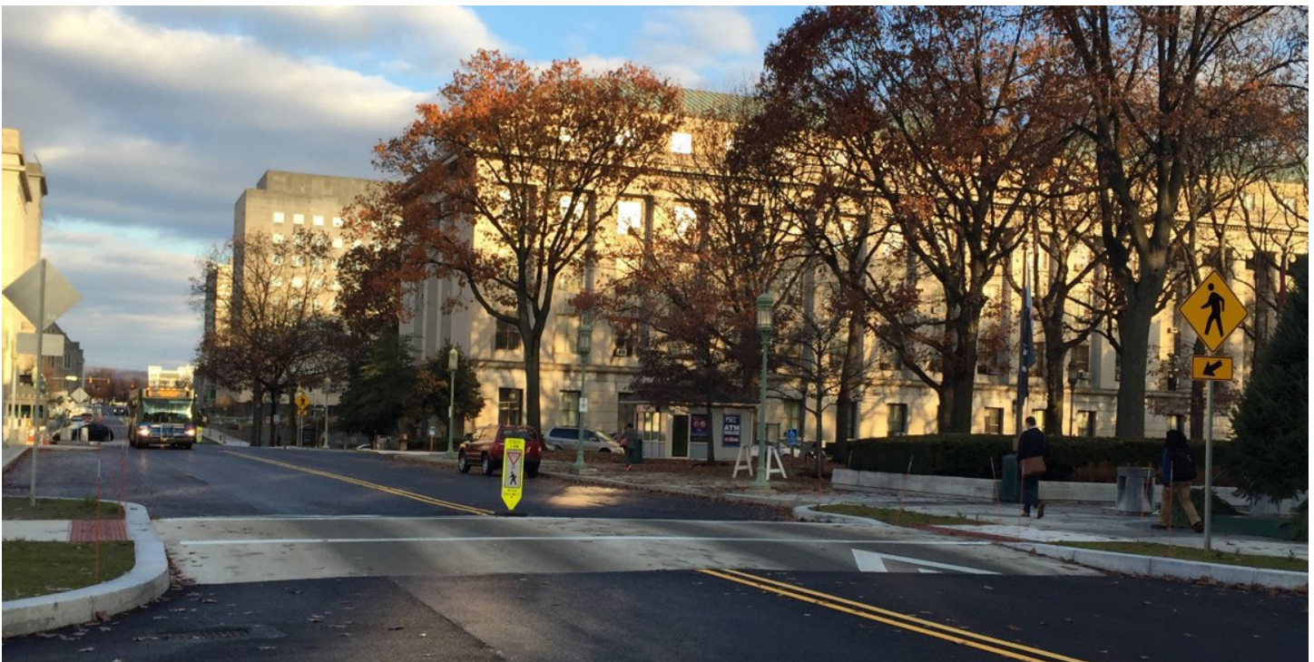
Figure 2. Raised pedestrian crossing with in-street signage. 1
